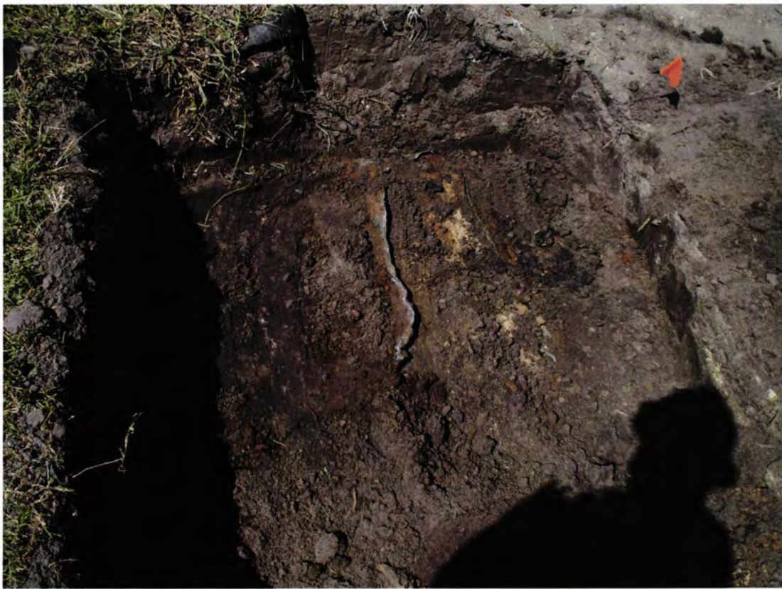
Picture 4: UST 767Althea-2 during excavation.
