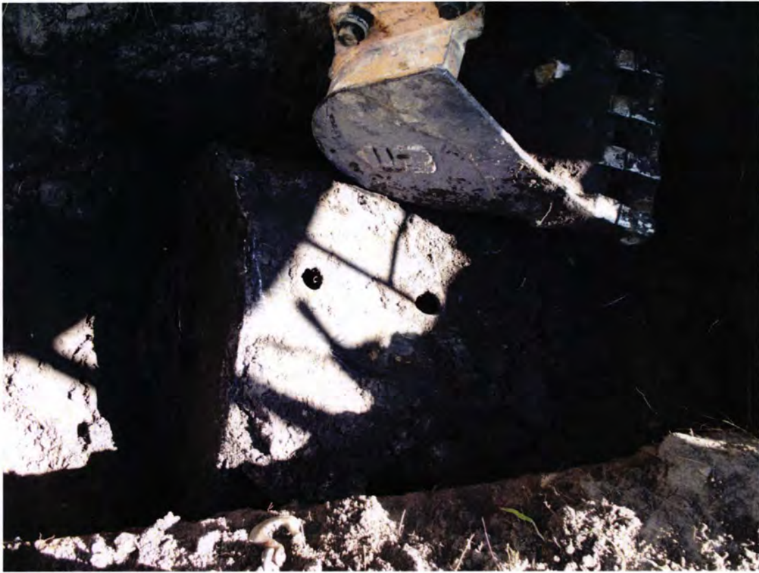
Picture 2: UST 767Althea-1 during removal.
